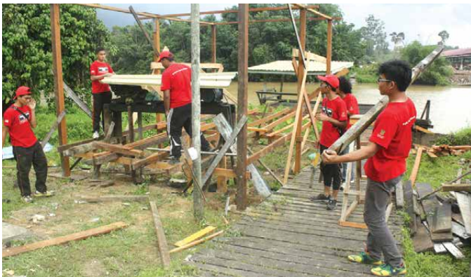
YSS student volunteers rebuilding a shelter for one of the generator sets in Kampung Labang, Bintulu
