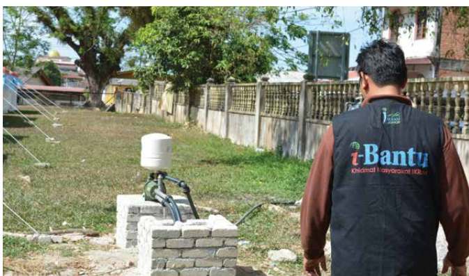
An i-Bantu worker shows off the water pump supply for the families at the shelter
