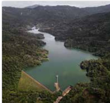
An aerial view of the Babagon Dam.
